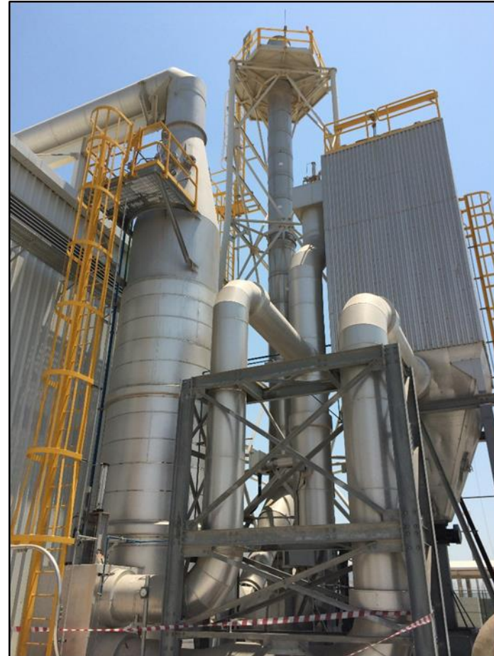
Evaporative Cooler with Dry Bag House Scrubber & Stack
