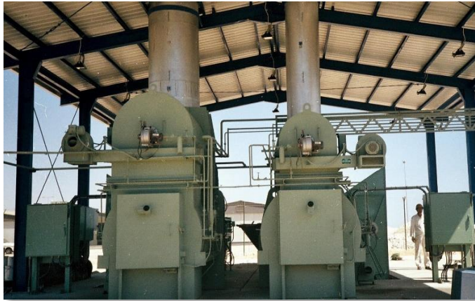
Outdoor Dual Reactor Combustion System at Jeddah Port Authority
