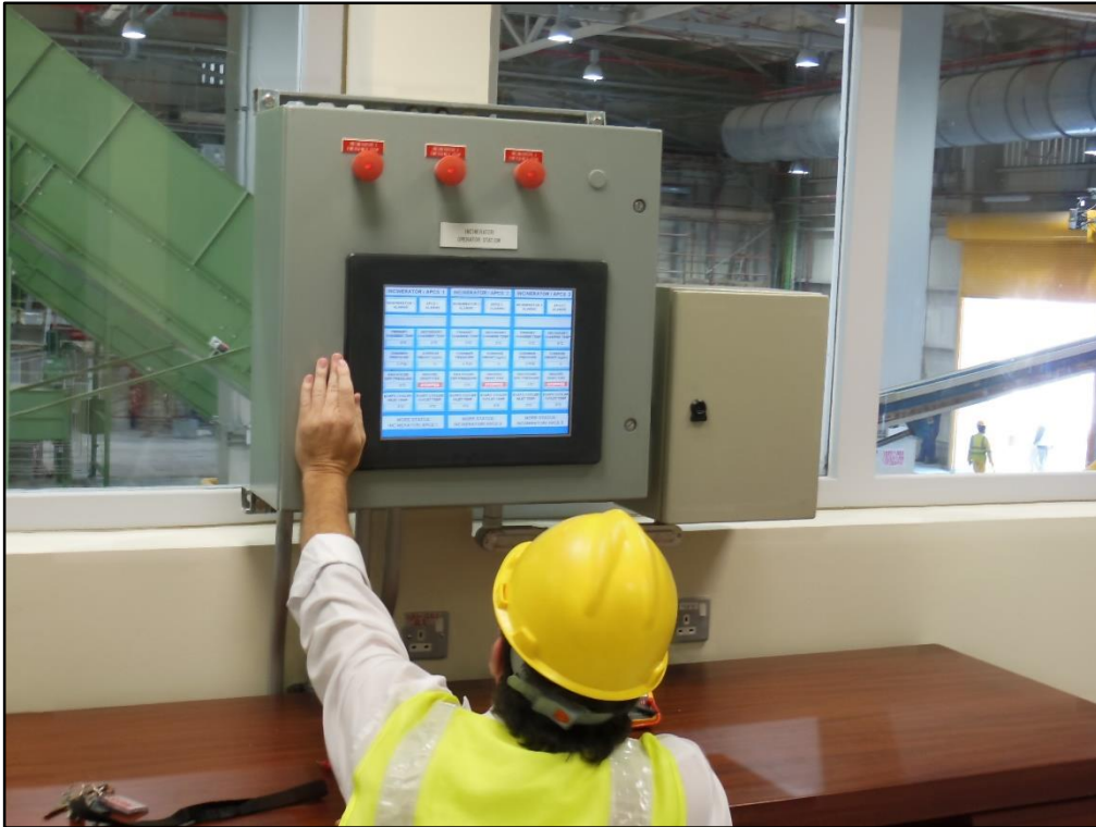
HMI (Human Machine Interface) Control Room Panel
